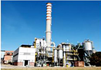
Paper&Pulp Bleach Plant
